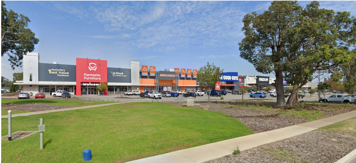
Image 1: view from William Street (northern side).
