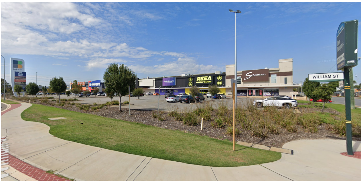
Image 2: view from William Street (western side).
